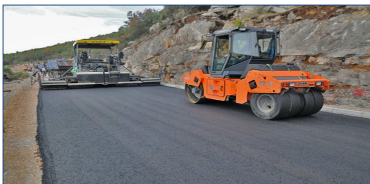
Image: Asphalt Resurfacing
