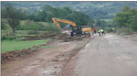
The construction site at the Tomaševo-Pavino polje road
