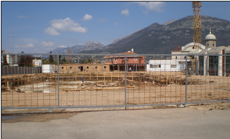
Construction site, May 2011
