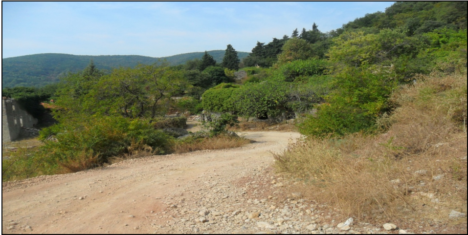
The allegedly finished road towards Krapina - a photograph taken in September 2012
