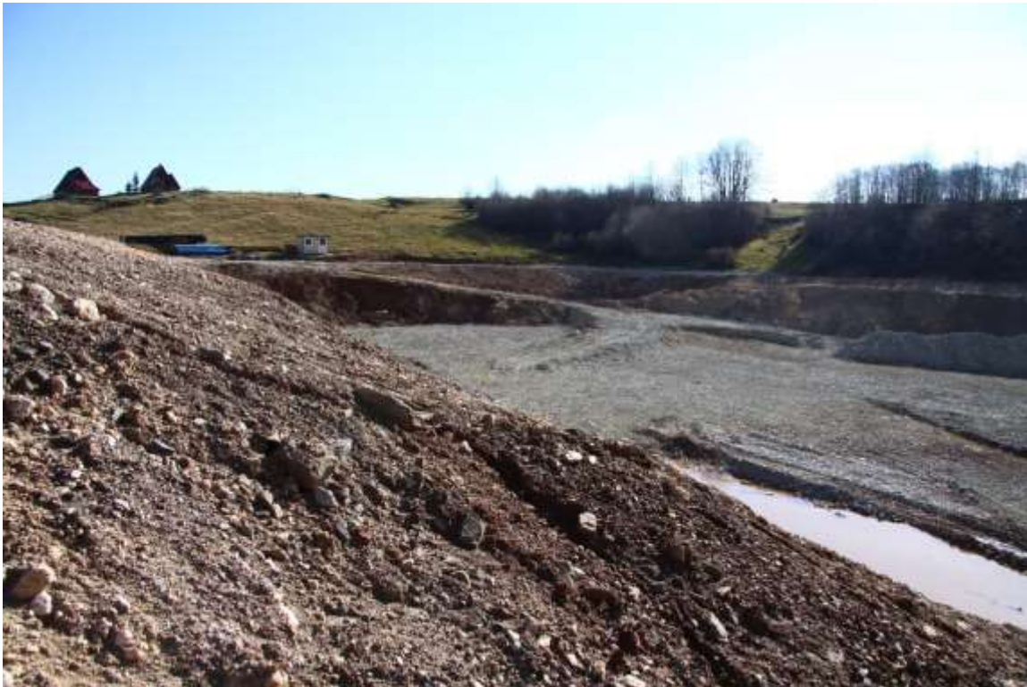
Figure 1: Water reservoir intended for the creation of artificial snow; Savin Kuk ski centre inside the World Heritage property
