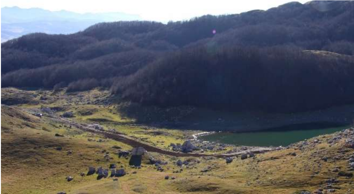
Figure 2: Newly constructed pipeline inside the property for feeding the reservoir in figure 1
