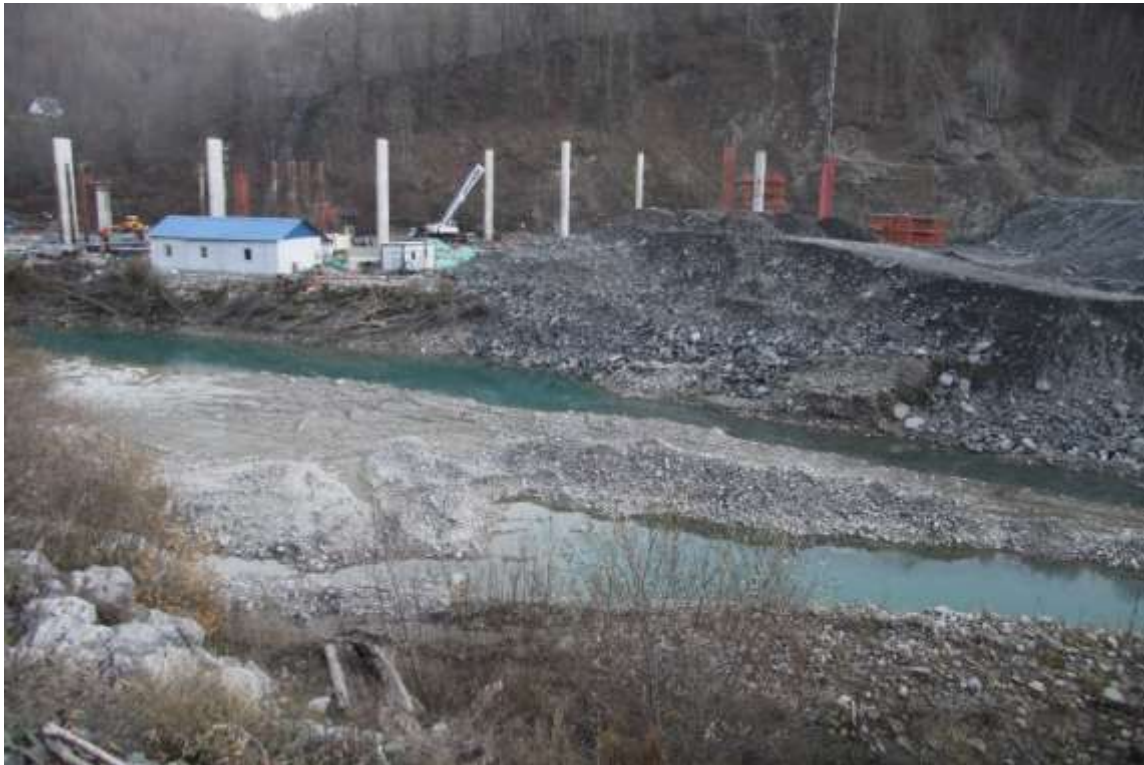
Figure 6: construction and deposition area in the floodplains of the Tara River
