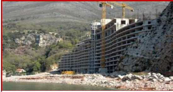
The facility under the first fix
